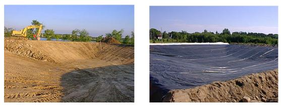
Dewatering is the result of physical separation according to the specific weight and evaporation of liquids (during a longer period). Removal of free liquids from the lagoon can easily be achieved with pumping from the surface while sediments can be removed by dredging or digging. Cleaning of the lagoons (sediment removal) is required in regular intervals.
