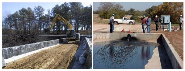
Drying beds are not particularly suitable for oily sludge's, as drying and draining are slow and the drain might be clogged with oil.
